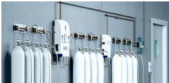
Medical gases buffer - manifold supply system
